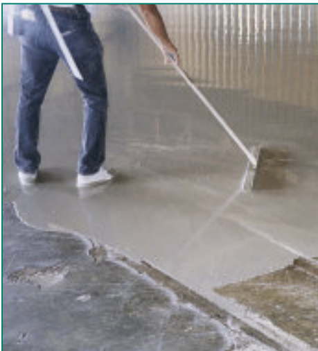
Level-Right makes this old, rough, pitted concrete floor smooth and level.
