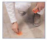
ON THE LEVEL — Maxxon applicators mark the floor with pins indicating the required pour depth. During the pour, Level-Right PLUS automatically flows to level, matching the height of the pins.
