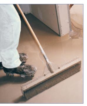
ROLLING WITH THE FLOW — A quick & easy roll is all it takes to finish a Level-Right PLUS application. Within an hour, light subtrades are back to work!
